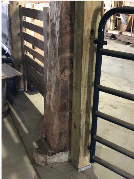
A tornado caused support posts to twist and shift, requiring additional support.
